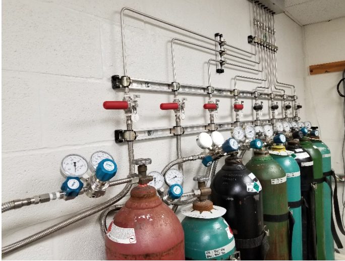
Figure 12: Fuel and Oxidizer Supply for Vitiated Heater
